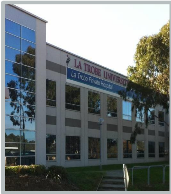
LaTrobe Private Hospital (VIC)
