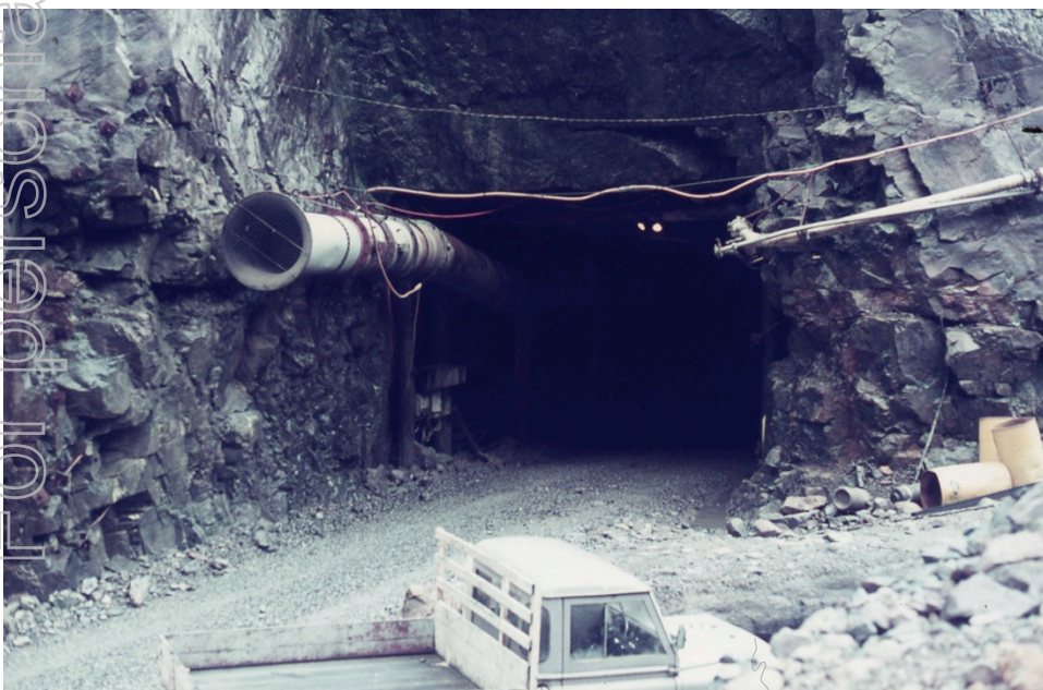
CLEVELAND MAIN PORTAL 1971
