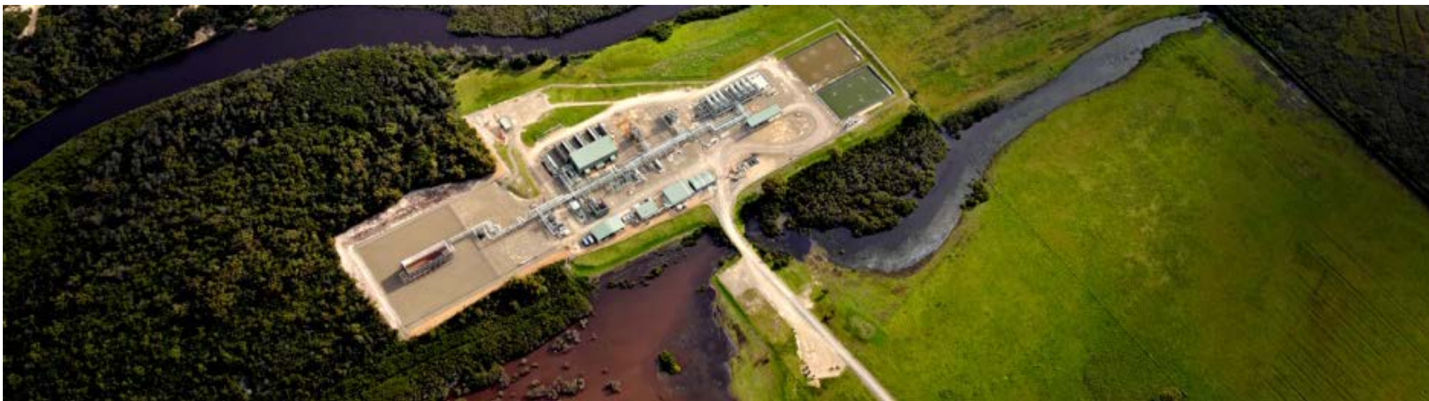
Orbest Gas Plant, hub for the Gippsland Basin Gas Projects
