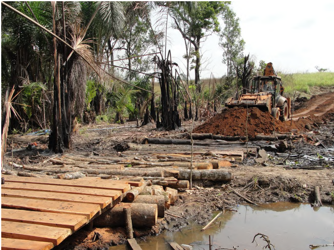
Figure 5: Access preparation across a swamp to reach Adoku workings.
