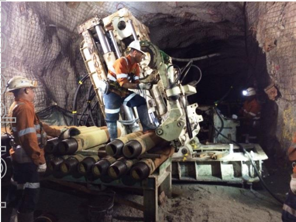
Bore hole machine in operation
