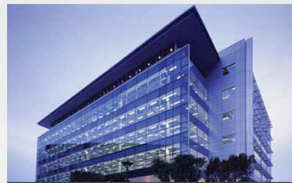
Building A, 1 Homebush Bay Drive, Rhodes NSW
