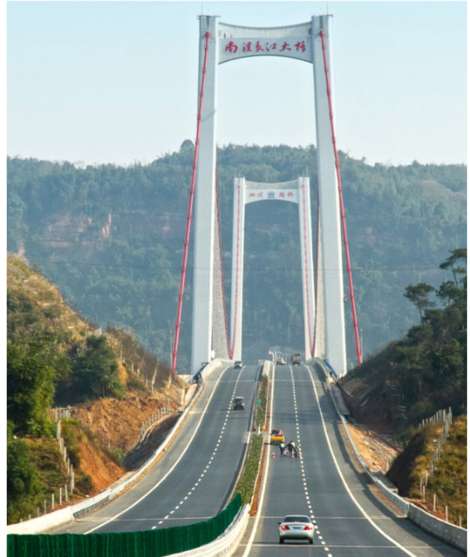
Yibin-Luzhou Highway built by SRIG
