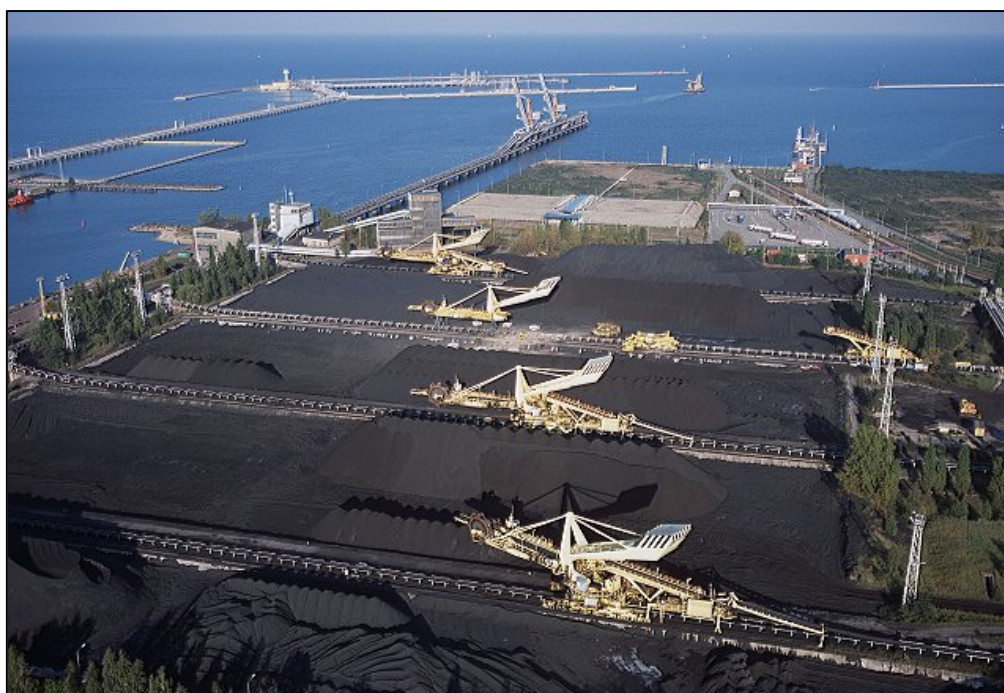
Figure 30: Gdansk Port – “Dry Bulk Terminal” – export facility stacker/reclaimers
