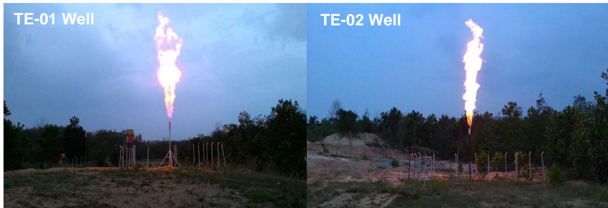
Gas produced circa 72 hours after dewatering commencement at site TE-01 and TE-02
