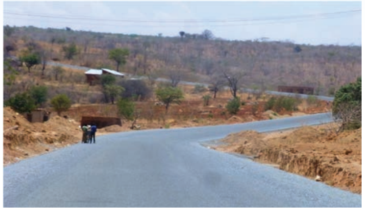
Figure 25: Upgraded bitumen road surface on the T8 east of Chunya, October 2013.
