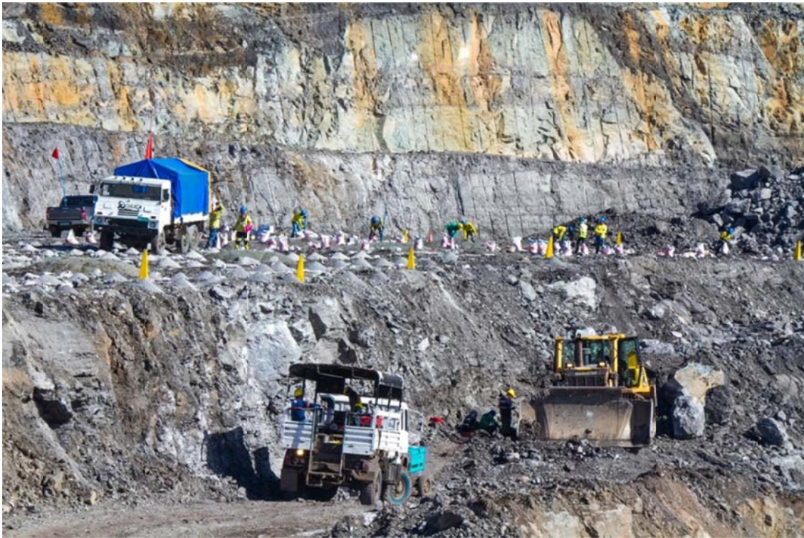
Figure 1: Mining Operation preparing for Drill and Blast
