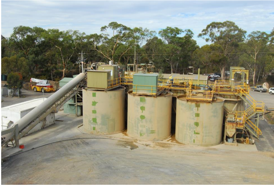
Figure 2. Operating Maldon Treatment Plant
