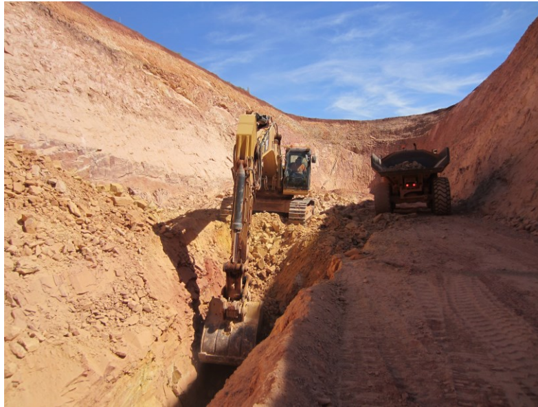
Excavating goodbye cut Western Limb Pit
