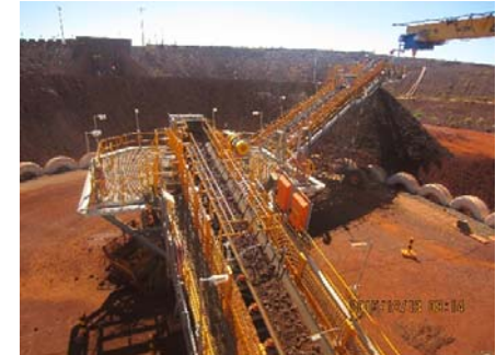
RCR supplied crushing plant at Rio Tinto's Mesa J mine, WA
