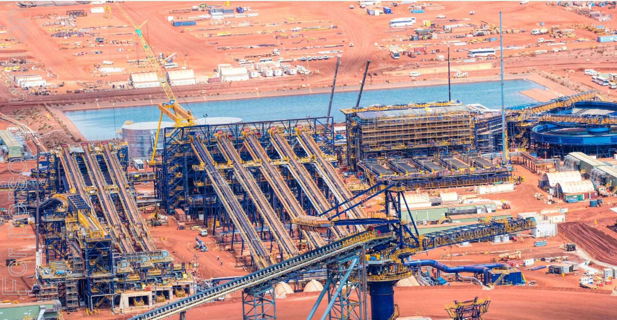
RCR SMP/E&I works at Roy Hill operations, WA
