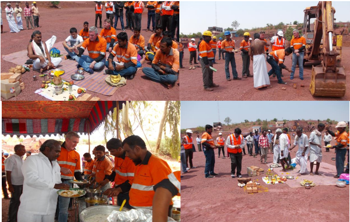
Puja Celebrations of breaking first ground for civil works
