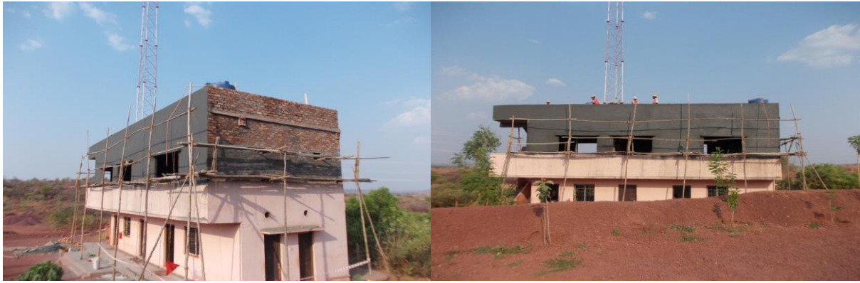
Office second story construction
