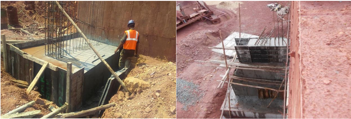
Retaining wall buttress construction
