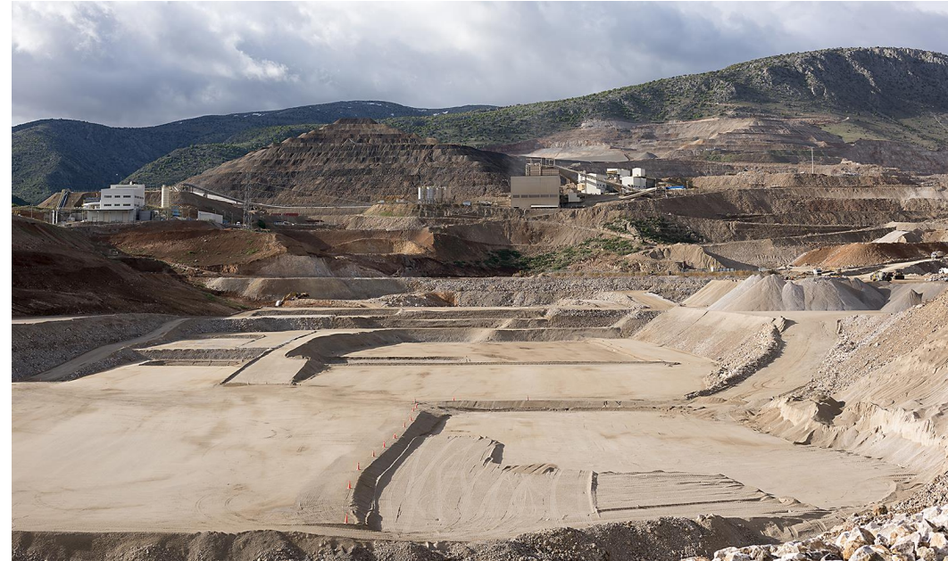
Sulfide Plant Site Earthworks
