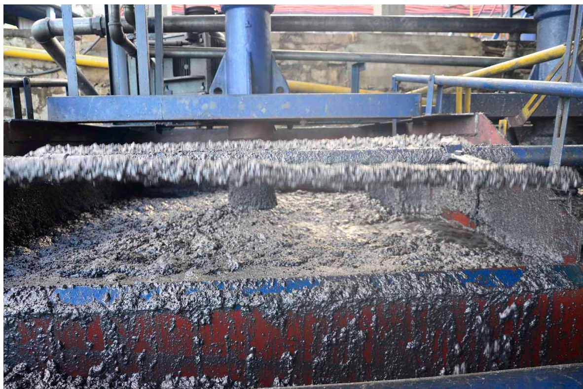
Figure 2: Graphite flotation at the Graphmada Processing Plant
