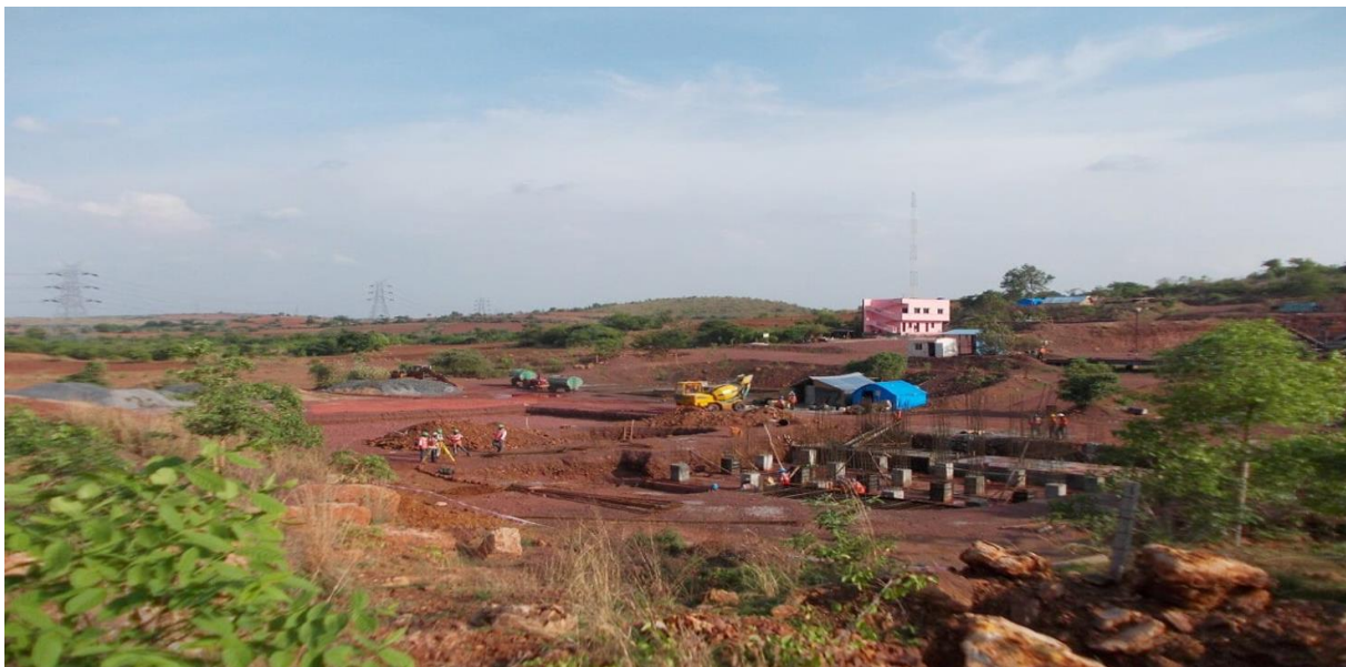
Foundation works concreting progression
