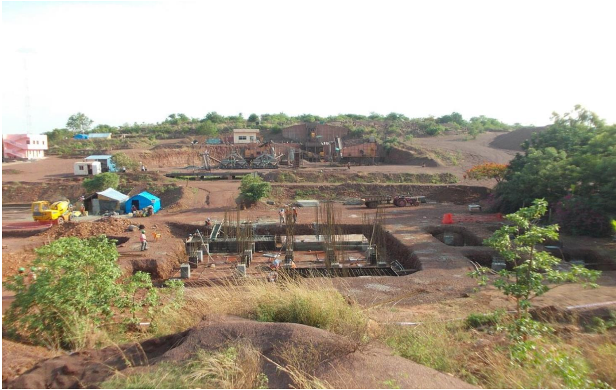
Foundation works concreting progression
