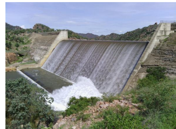
Top Up Dam – connected to site by Genex pipeline (overflowing in 2015 wet season)
