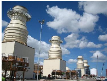
Open Cycle Gas Turbines
