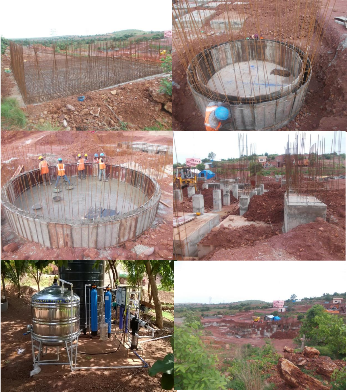
Backfilling and foundation works with Reverse Osmosis drinking water equipment
