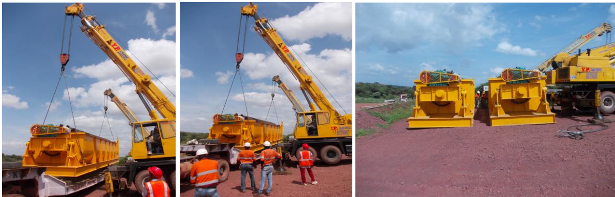
Classifier equipment arriving on site
