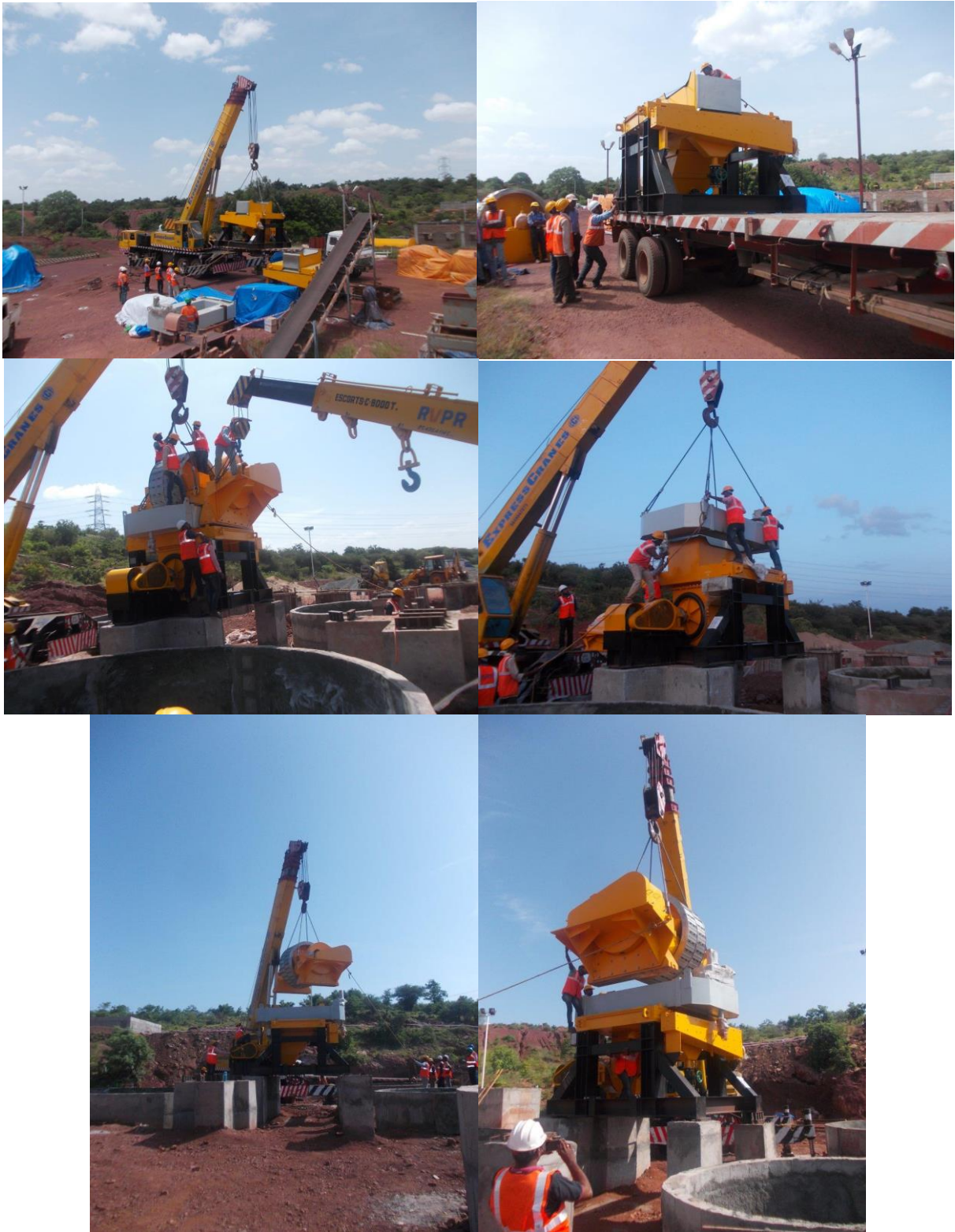
WHIMS Number One Erection
