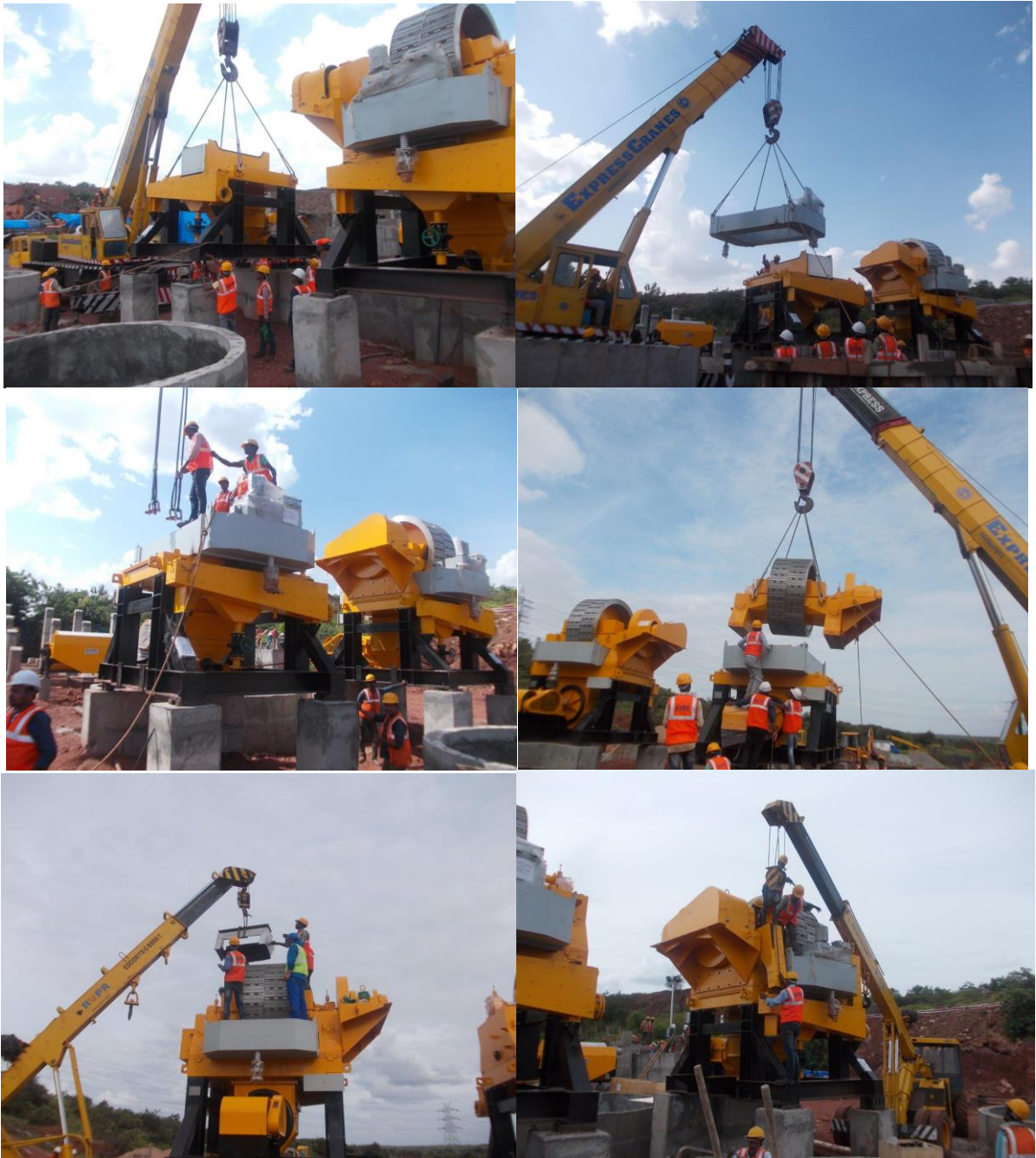
WHIMS Number Two Erection
