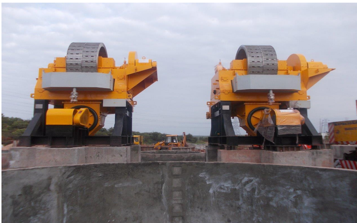
The Two WHIMS Safely in Place
