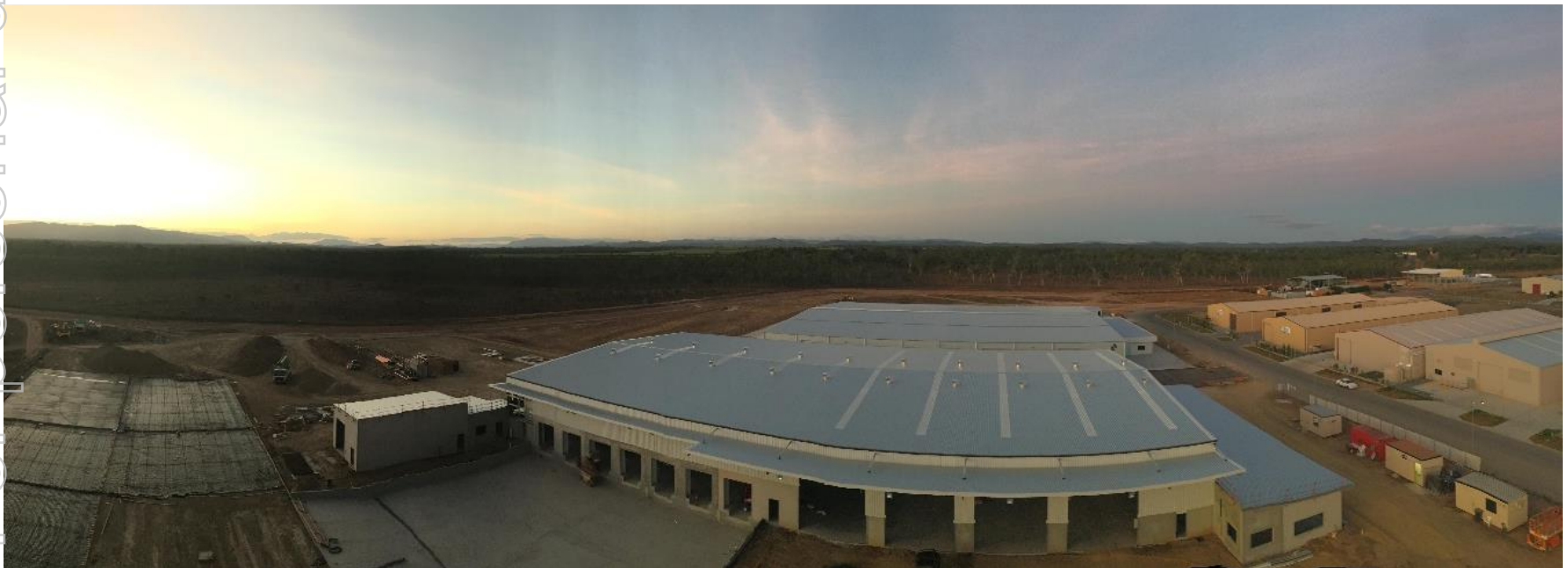
Mareeba depot near completion
