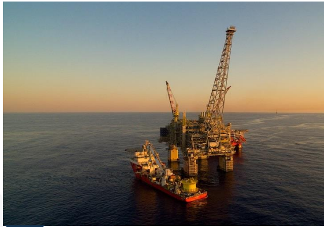
Wheatstone Offshore Platform Client: Chevron & BAE Systems
