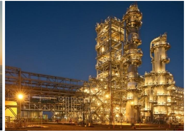
Karratha LNG Woodside Client: Woodside Petroleum
