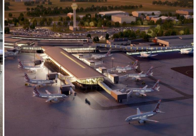
Perth Airport T1 & T2 Client: CAM and Vodafone
