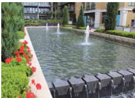
Hydroxypure water feature, London.
