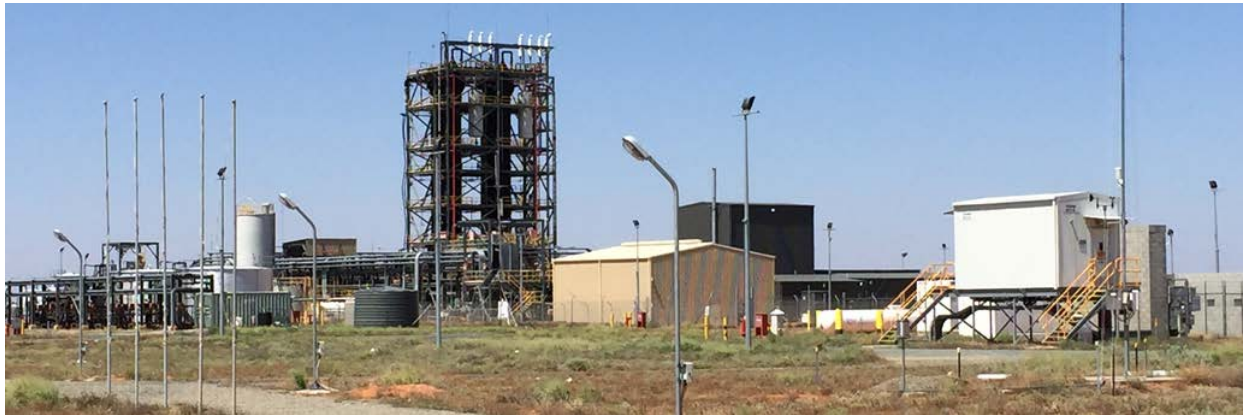
Figure A1: Honeymoon Uranium Process Plant
