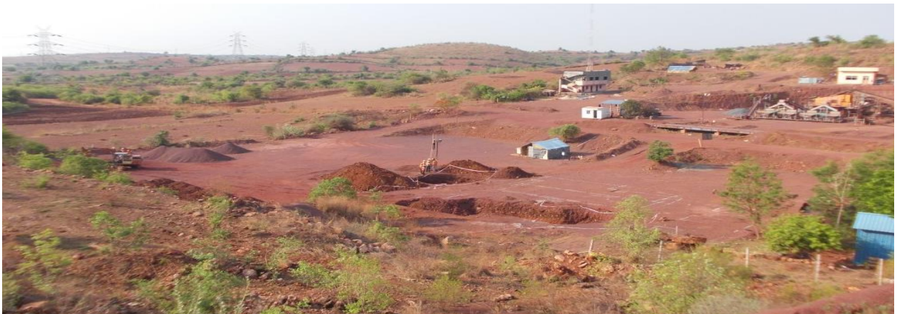
Sequential Site Images Showing Construction Progress
