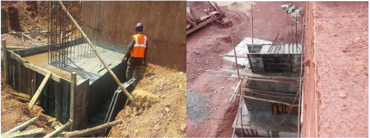
Retaining wall buttress construction
