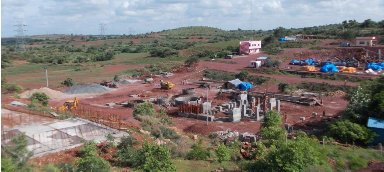
Sequential Site Images Showing Construction Progress
