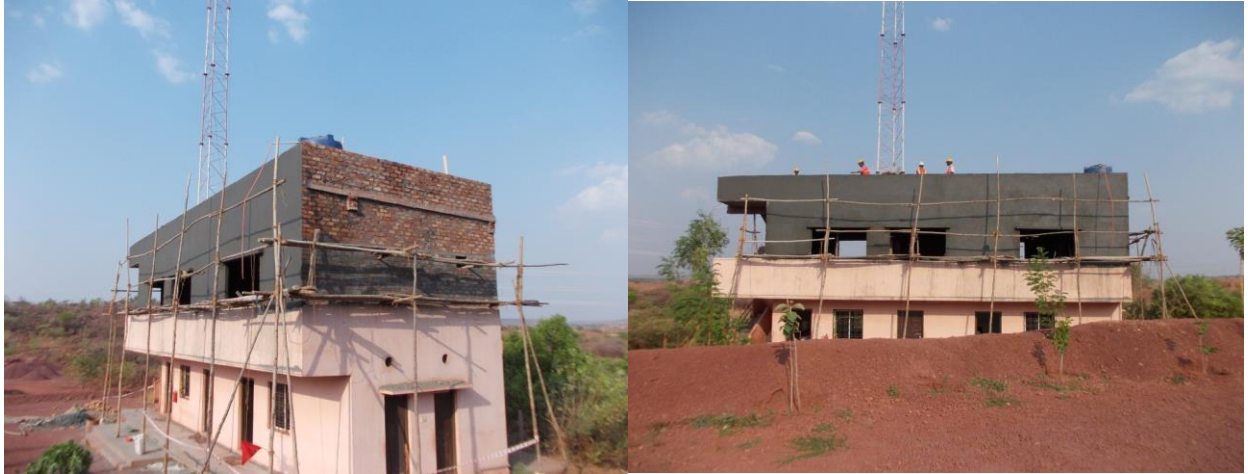
Office second story construction
