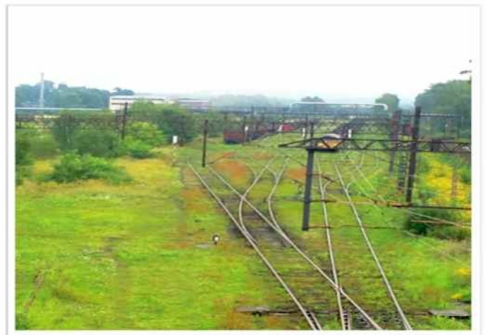
Figure 4 – Railway Siding at Debiensko
