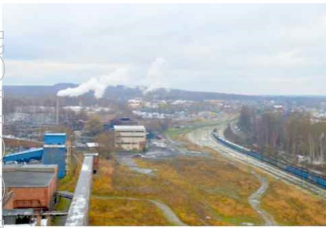
Figure 3 – Existing Site Facilities
