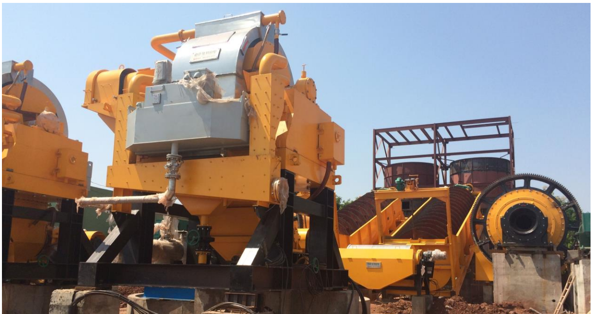
Final Fitout of Chinese Equipment
