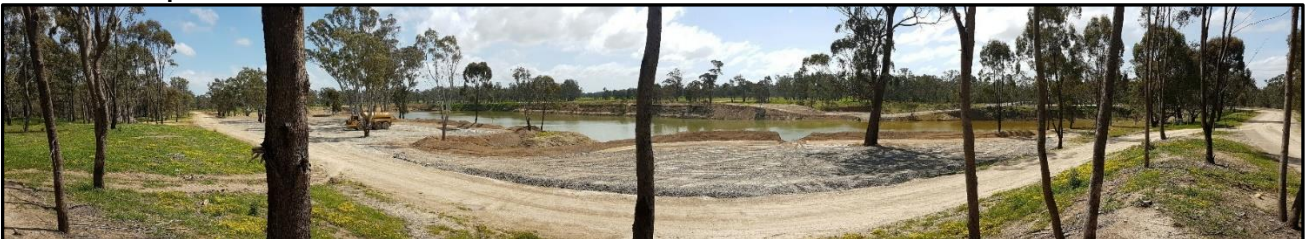
Photo 2 Preparation for West Pit Rehabilitation
