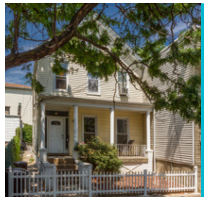
Recently acquired 31 Sherman Avenue, Jersey City Heights
