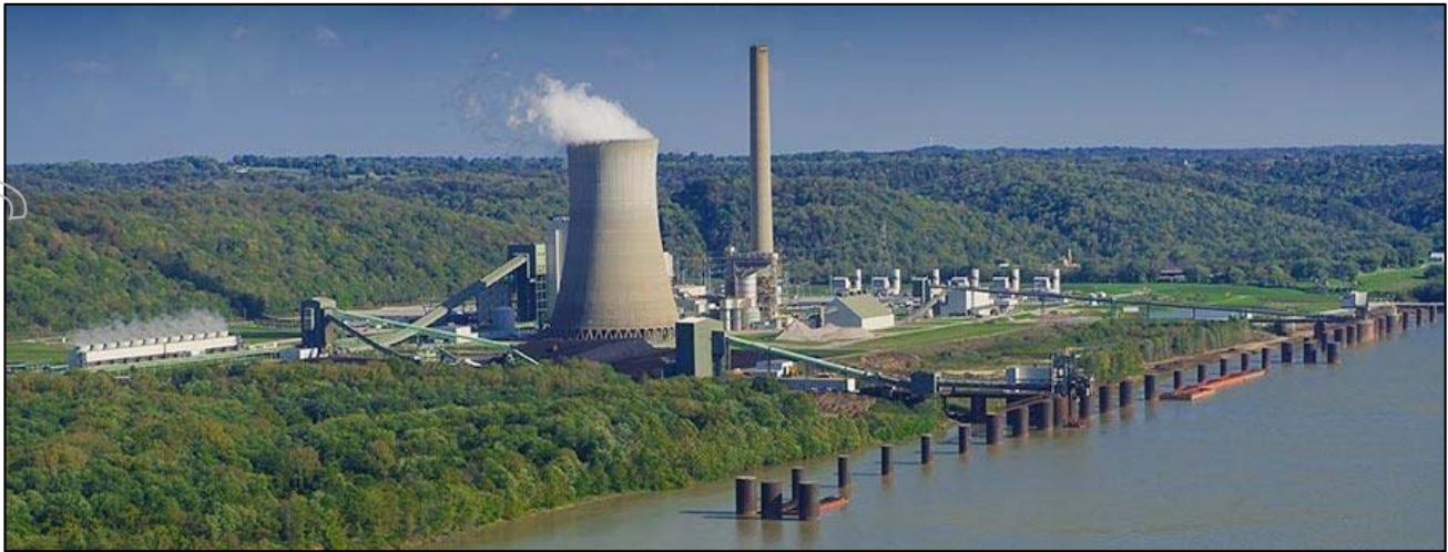
Figure 17: LG&E and KU's Trimble County Power Plant on the Ohio River
