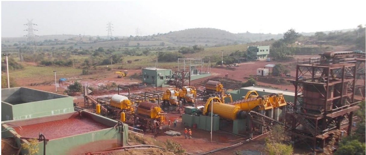
Wet plant overview
