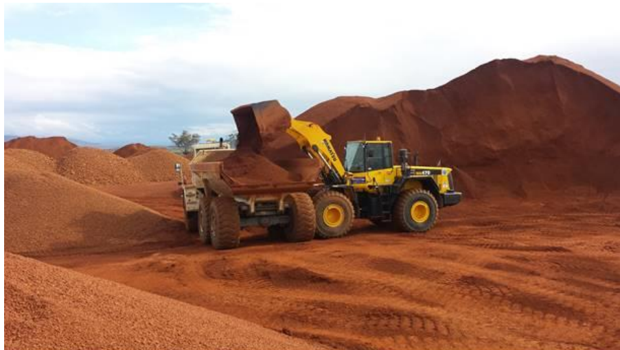
Figure 5 Blending 35,500 tonnes of cement-grade bauxite at Bald Hill Mine Site
