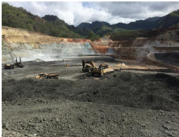
Image 1 – Excavating blasted material in Kali Kuning pit
