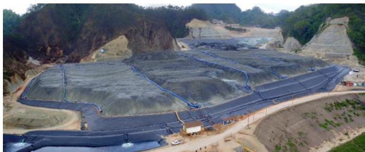
Image 3 – Stacked tonnes on KKV Leach Pad
