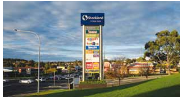
Shellharbour Retail Park
