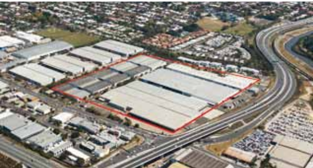
Hendra Distribution Centre
