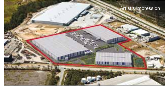
Yatala Distribution Centre
