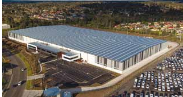
Ingleburn Distribution Centre
