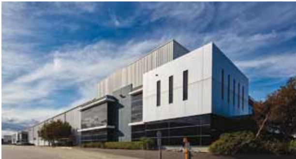
20-50 and 76-82 Fillo Drive and 10 Stubb Street
