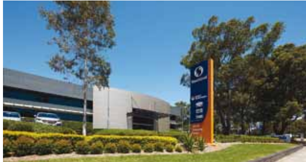
Macquarie Technology Centre
