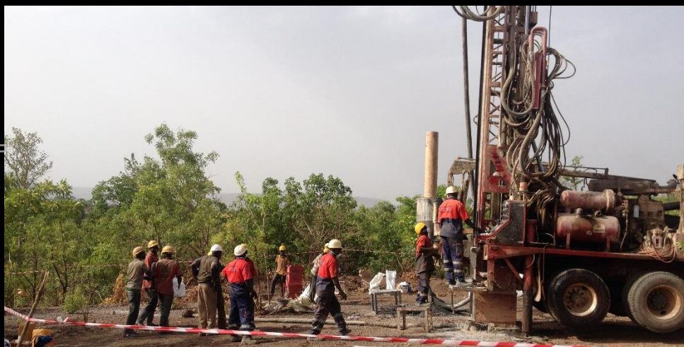
READILY ACCESSIBLE DRILL RIGS AND EQUIPMENT
