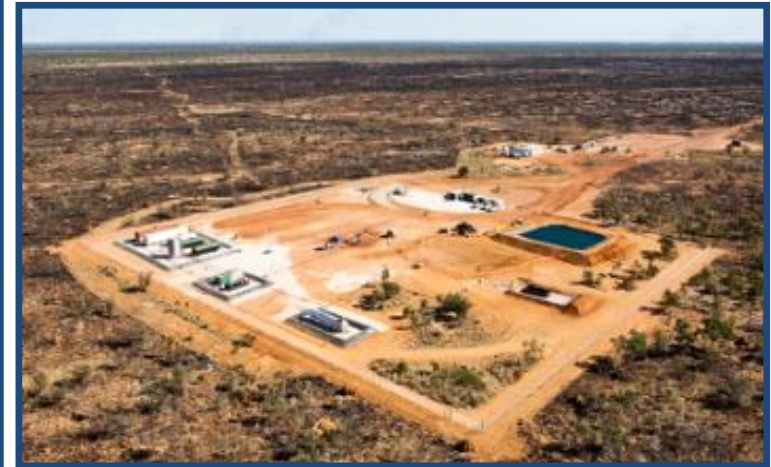
Ungani field facility
