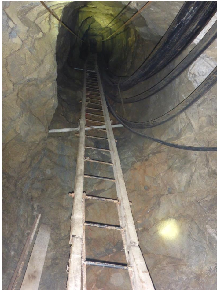
Figure 10. Air Leg Access Rise up to the 1465-8764 Stope at the A1 Mine
