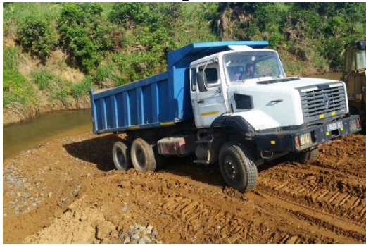
Photo 3 – River crossing construction
