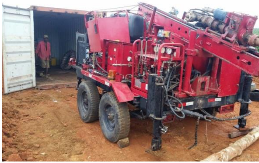
Photo 1 – Drill Rig on arrival
