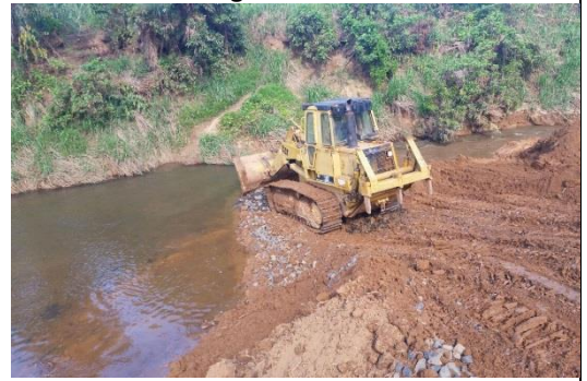
River crossing construction
