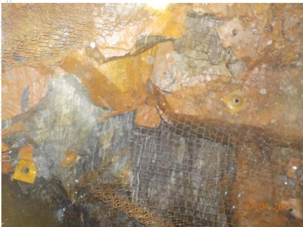
Typical ground support mesh and bolting in Shaft H.
