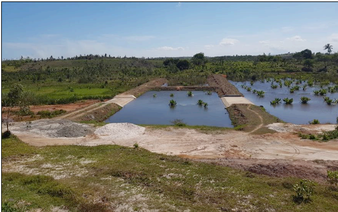
Figure 8 – Cleaner dams, part of the long-term tailings storage management at Graphmada.
