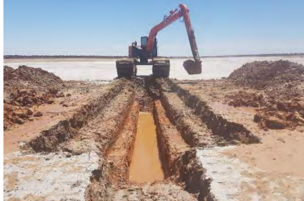
Photo: Trench excavation at Lake Wells 1 Significant trenching required to access low grade brines
