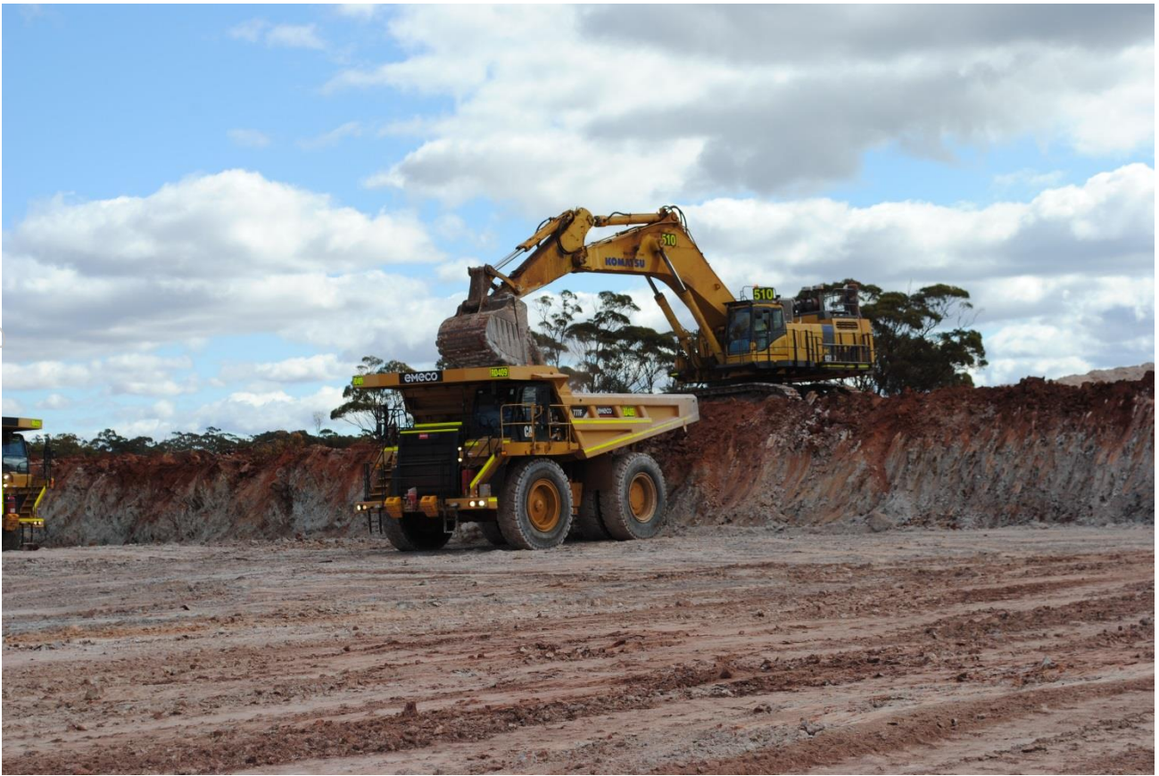
Excavating and loading waste at Penny's Find Project
