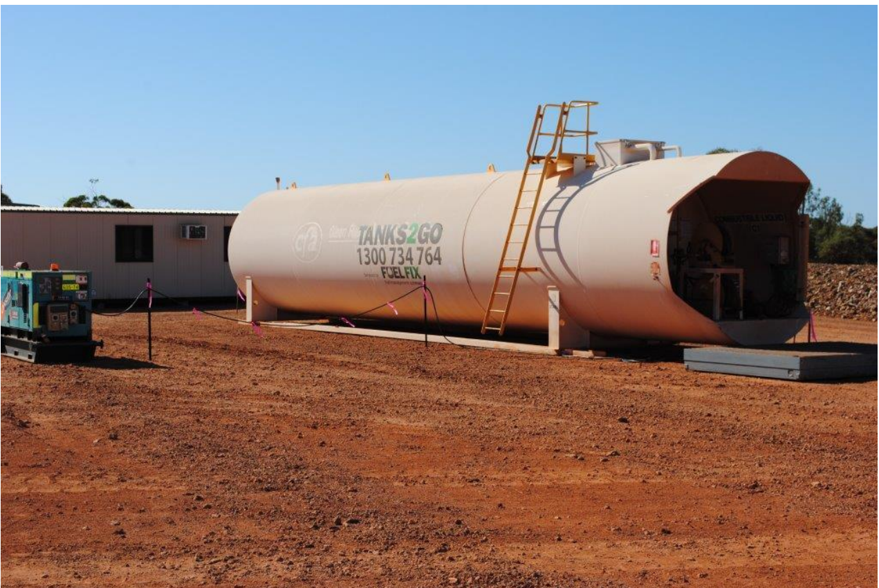
Self bunded fuel tank being installed at Penny's Find
