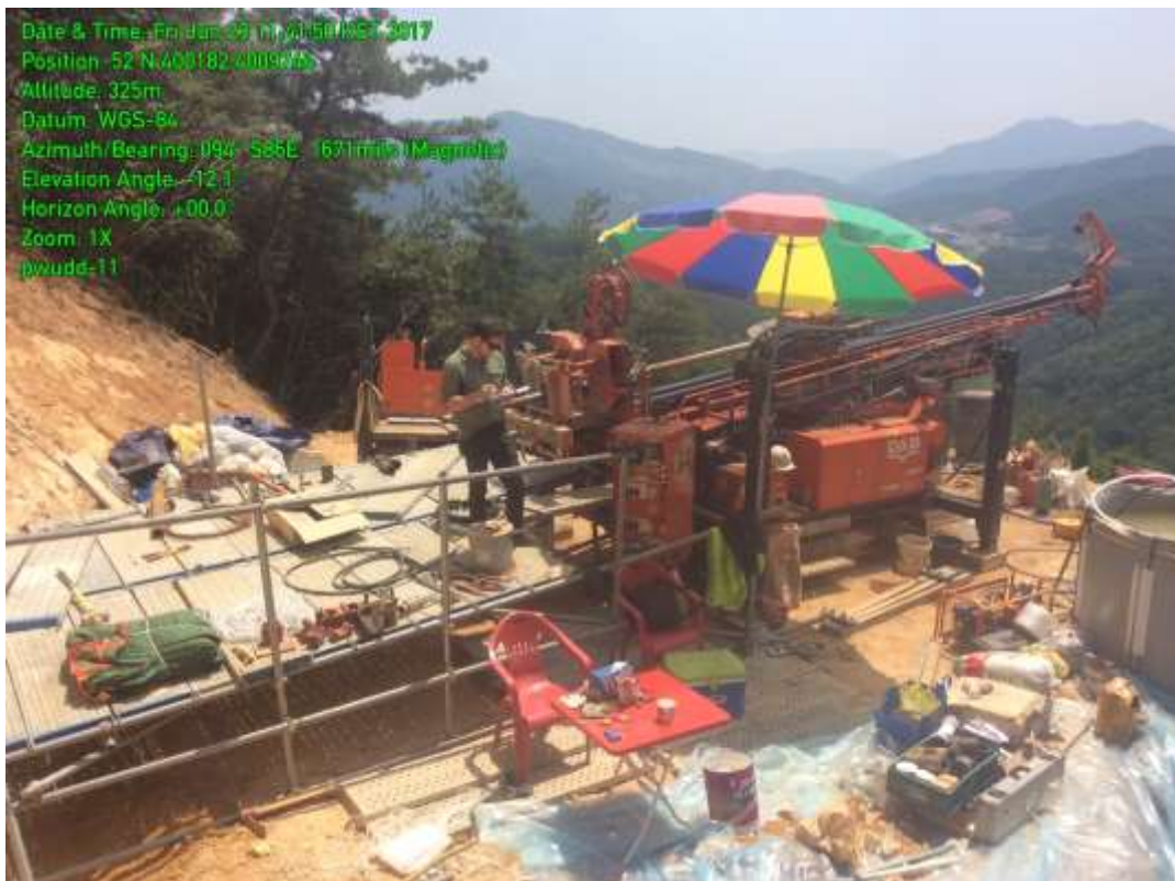
Photo 6. Sub-horizontal drilling into the mountain, Weolyu South, SK
