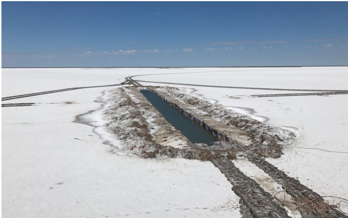
Figure 3. Construction Completed at T16
