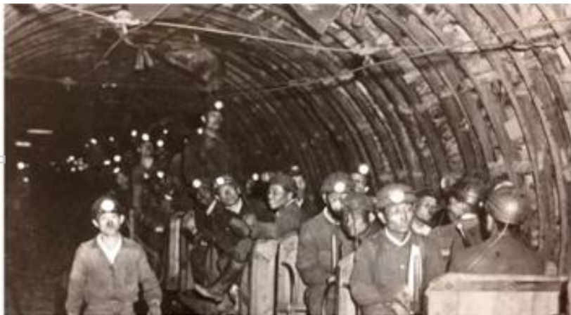
Inside the main adit
