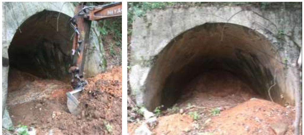
Photo 1 and 2: The entrance to Decline Shaft being excavated.
