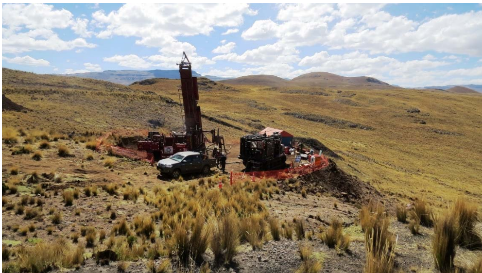
Figure 2 - Drilling at Platform 8 (BEP8) Outside Resource Shell
