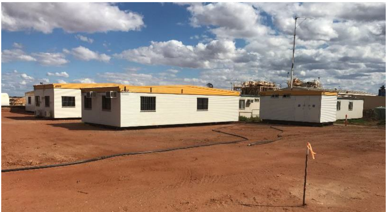
Figure 7 | New site offices in position
