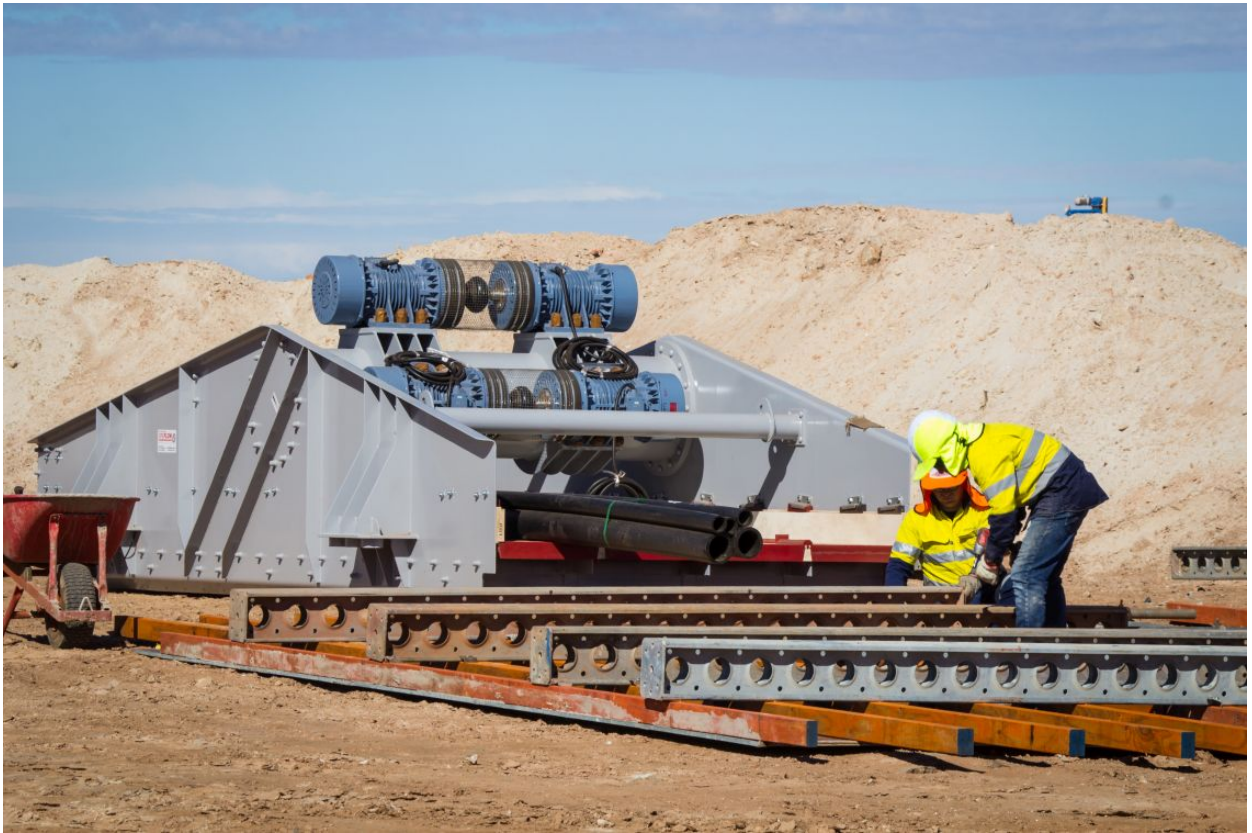
Figure 2 | First screen being delivered to Bald Hill site
