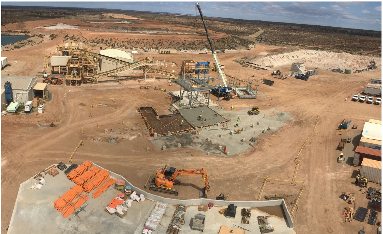
Figure 1 | Bald Hill project construction aerial view (September 2017)
