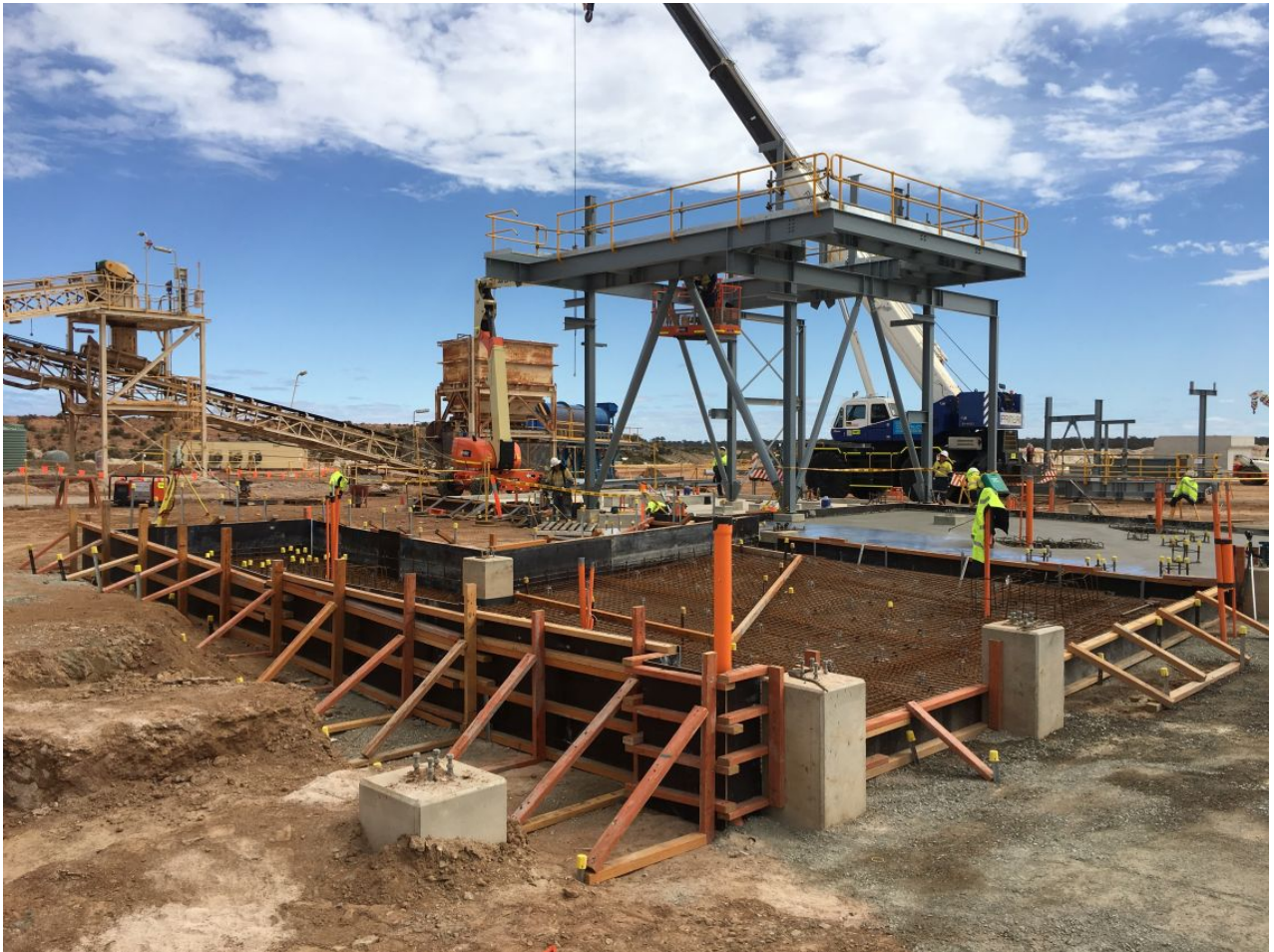
Figure 6 | Structural Steelwork being erected
