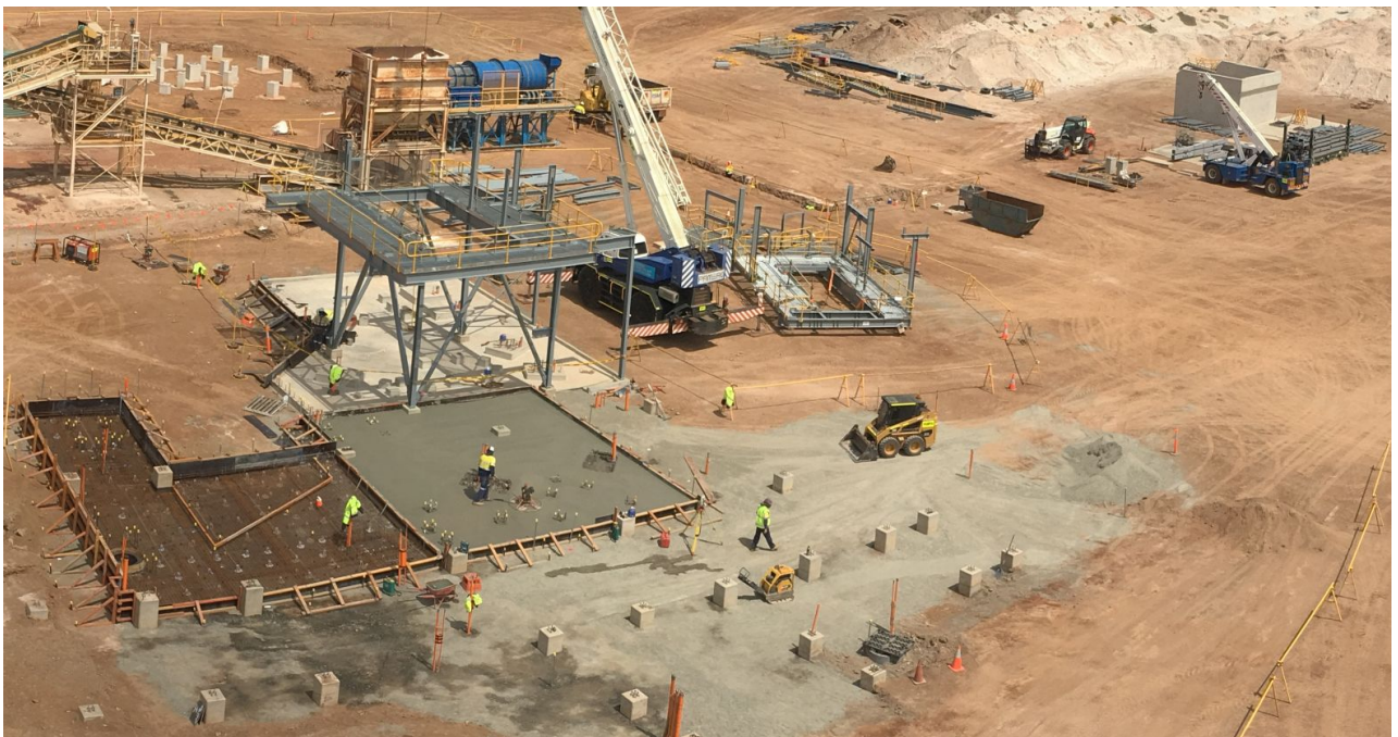
Figure 5 | Feed Bin Wall & Concrete Footings completed
