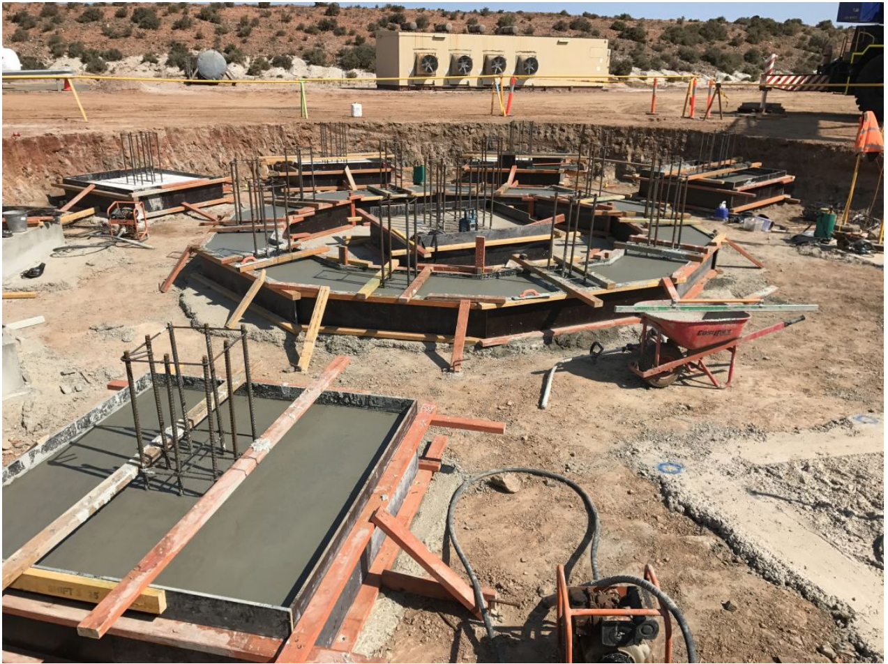
Figure 4 | Concrete works for Thickener
